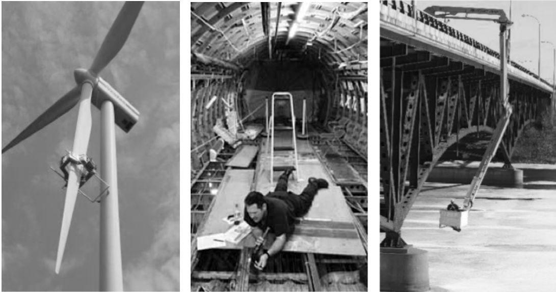
(a) Wind turbine inspection (photo courtesy of Kaufer online). (b) Aircraft fuselage inspection (photo courtesy of Sandia National Lab., USA). (c) Bridge inspection (photo courtesy of Aspen Aerials, USA).
