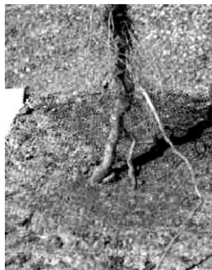
Fig. 2.13 GCL damaged caused by roots (after Mazzieri and Pasqualini, 1997)
