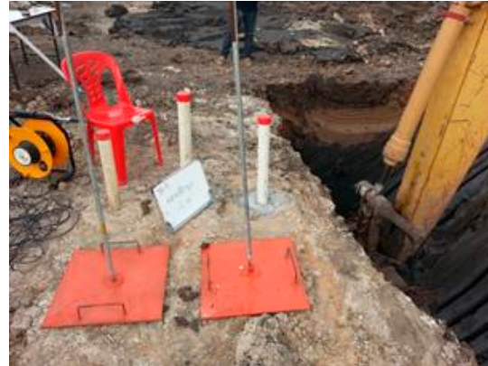
Fig. 11. Installation of the surface settlement plate behind the soil cement wall.
