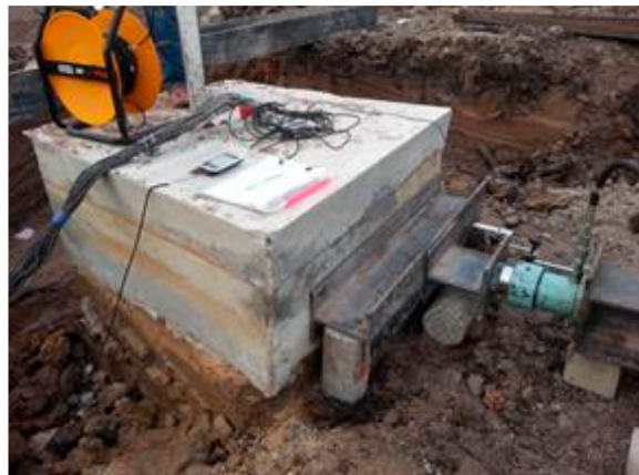
Fig. 21. Horizontal load test setup.
