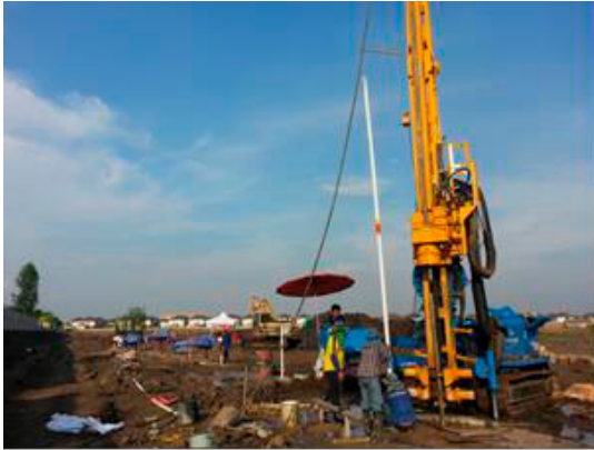
Fig. 10. Installation of the inclinometer with diameter of 70 mm.
