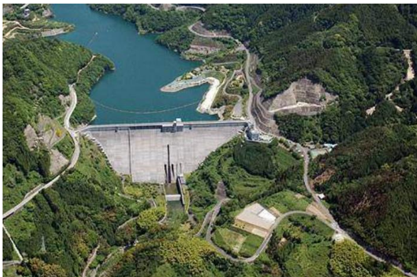
Figure 3.10: Kyuragi dam (Source: MLIT Takeo office, 2011)
