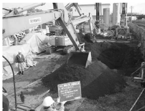
Photo 27 Backfilling of the insolubilized soil
