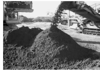
Photo 13 Improved embankment soil
