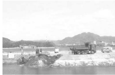
Photo 9 Backfilling by backhoe
