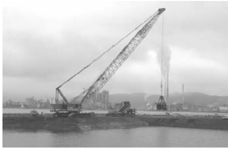
Photo 8 Backfilling by clamshell
