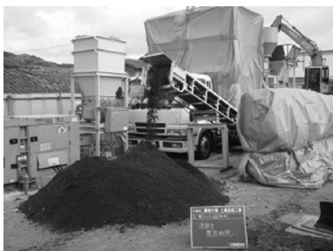
Photo 26 Output of the improved soil
