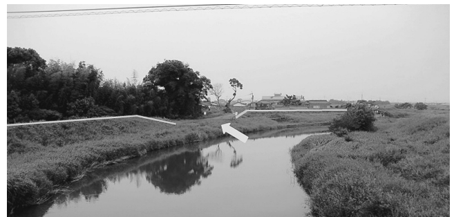
Fig.2 Overflow embankment of the Jobaru River (Tsurunishi District, Kanzaki City, Saga Prefecture)
