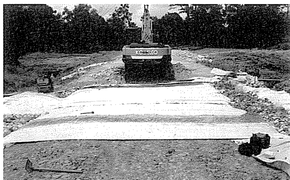
Fig. 4 Completion of prestressing work on geosynthetic reinforcement (after Chew et al. 2005)
